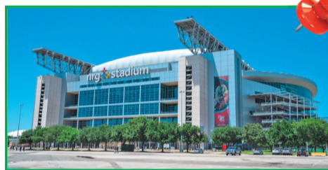
NRG STADIUM - HOUSTON
