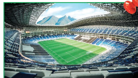
METLIFE STADIUM - NEW JERSEY
